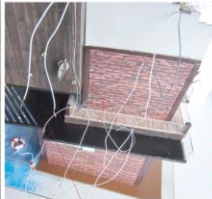
Grey line extension cord of the second floor
